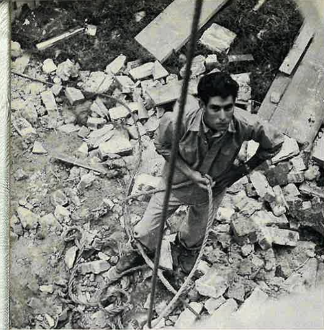
The old walls come down . . .
